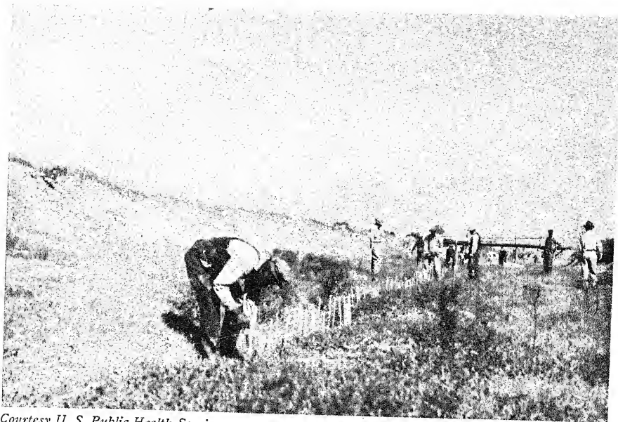
Figure 25. Setting out dynamite charges to deepen an existing drain by blasting
